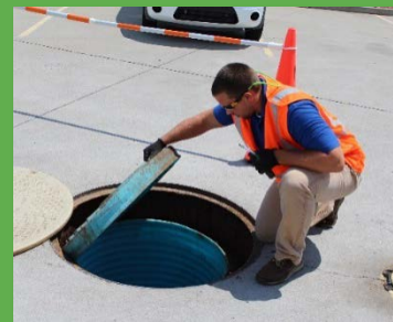
Inspecting a containment sump
